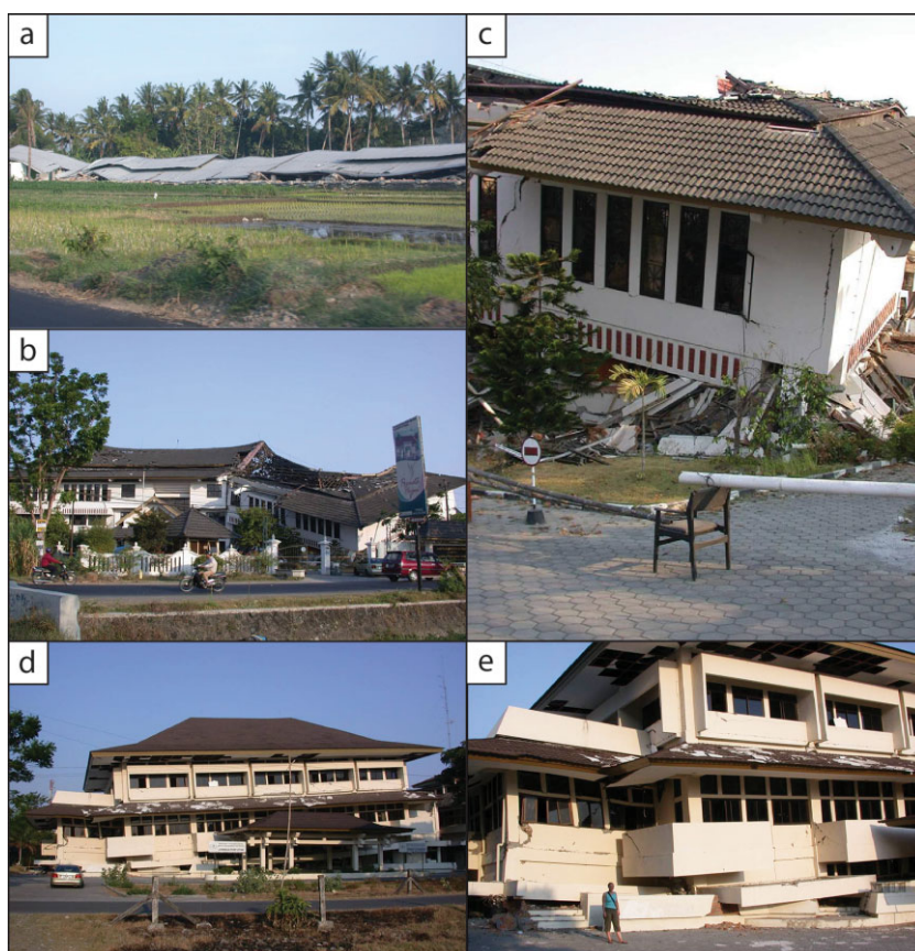
Fig. 10. Damage caused by the 2006 earthquake in Yogyakarta city and surroundings. (a) Collapsed building south of Yogyakarta. Note the roof rests on the ground, i.e. the walls have collapsed entirely. (b, c) Building of the governmental financial and development agency in Parangtritis Street (Jalan Parangtritis). (d, e) Damaged building of the Department of National Education, Institute of Art of Indonesia, Gadjah Mada University.
