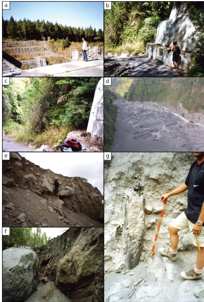
Fig. 8. Hazard mitigation. (a) Example of a Sabu dam on the slopes of Merapi. The Sabu channel system aims to confine lahars and pyroclastic flows and creates artificial basins to trap material that is moving downhill. (b, c) Early warning system in steep valleys on Merapi's higher slopes. An electric signal is sent if the steel rope is disturbed. (d) Sand mining creates sediment traps in recent BAF deposits on the medium altitude slopes of Merapi. (e–g) Impression of recent BAF deposits from Merapi. Note the mixture of large blocks and fine ash plus entrained debris like charcoaled tree trunks.
